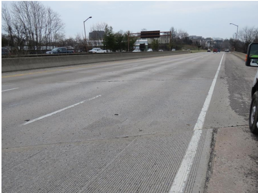
VIEW ACROSS TOP OF WEARING SURFACE
