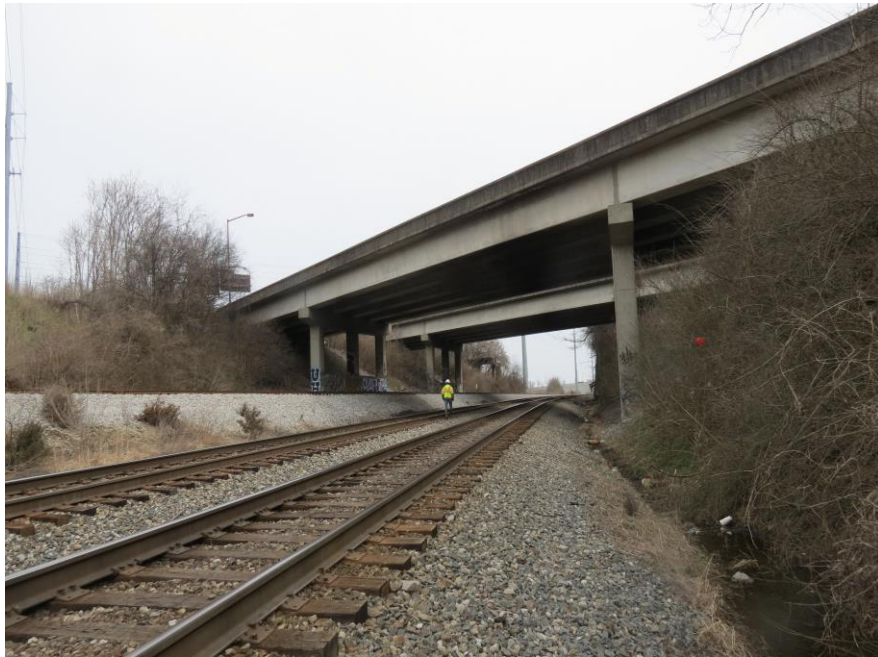
CLEARANCE VIEW RT. SIDE
