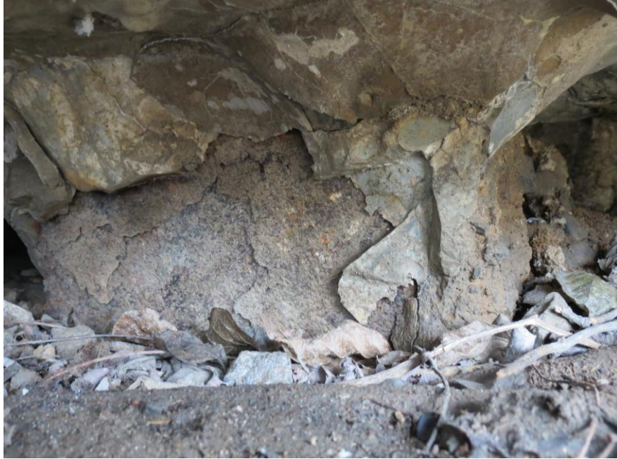
EXP. PILE AT ABUT. #2
