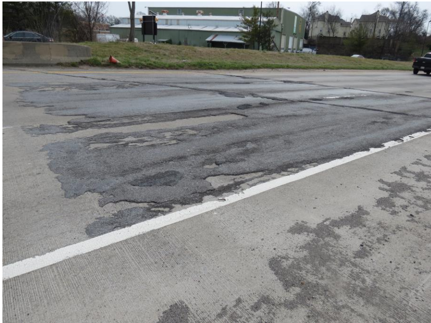
WEARING SURFACE SP. #3 W/ ROUGH A/C , SCALE
